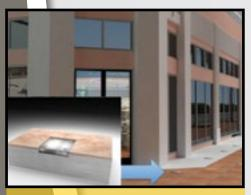
Post inserts are covered over with plates in the side walk. Plate could also be designed to aesthetically disappear.
